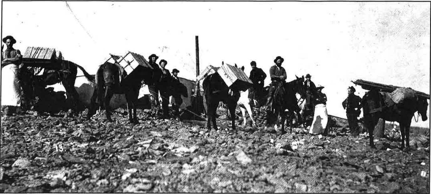
Triangulation party on Uncompaghre Peak, Colo., 1895, site of one of the longest network lines ever established—183 miles.
