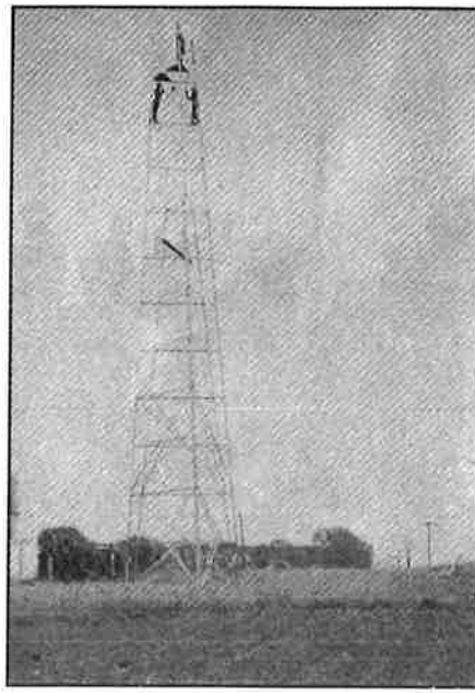
Towers of wood (left) reached only about 50 feet. Metal towers (right) designed by Bilby reached over 100 feet.
