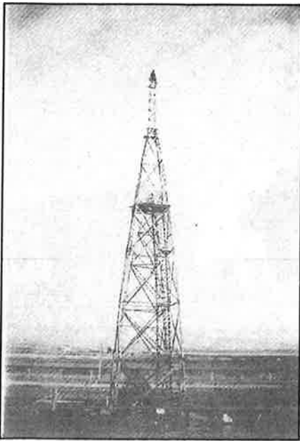
Towers of wood (left) reached only about 50 feet. Metal towers (right) designed by Bilby reached over 100 feet.
